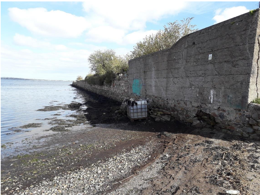
Plate 4.27 Existing Sea Wall – Northwest edge
