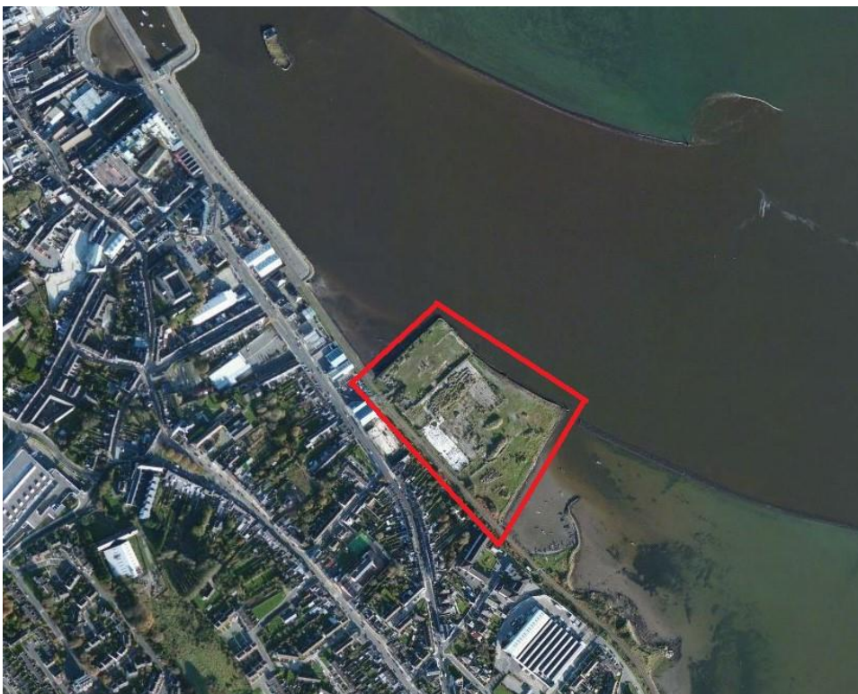
Figure 1. Trinity Wharf, Wexford, showing location
