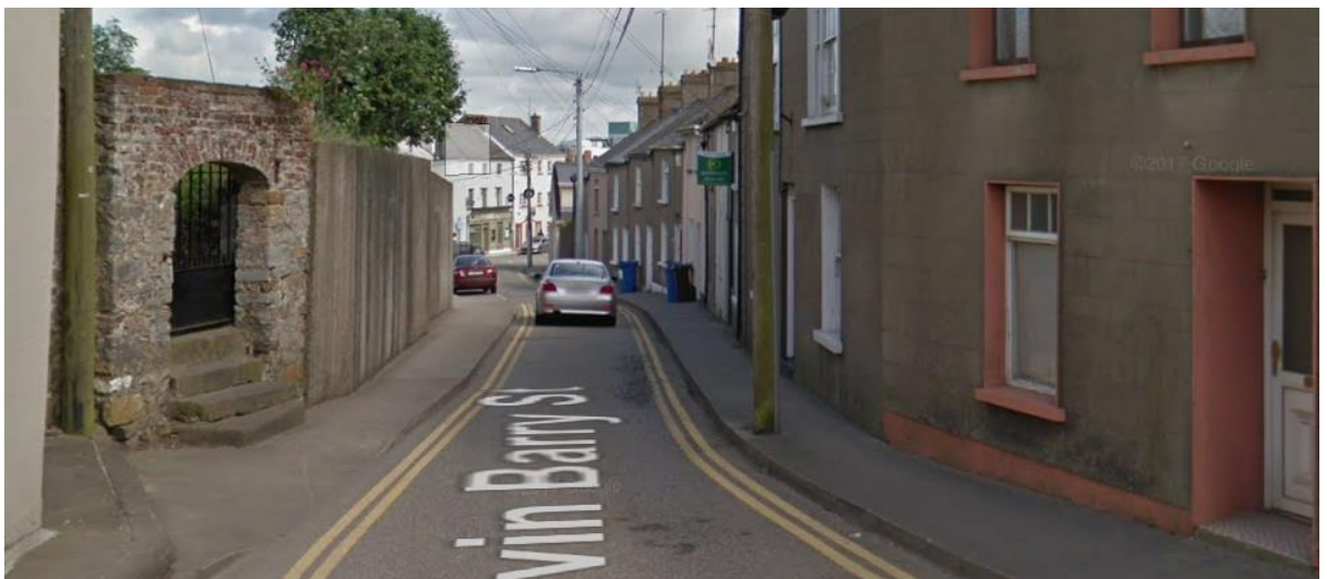
Figure 9- Kevin Barry Street – Note: narrow one-way street lined by high/medium density housing on one side.
