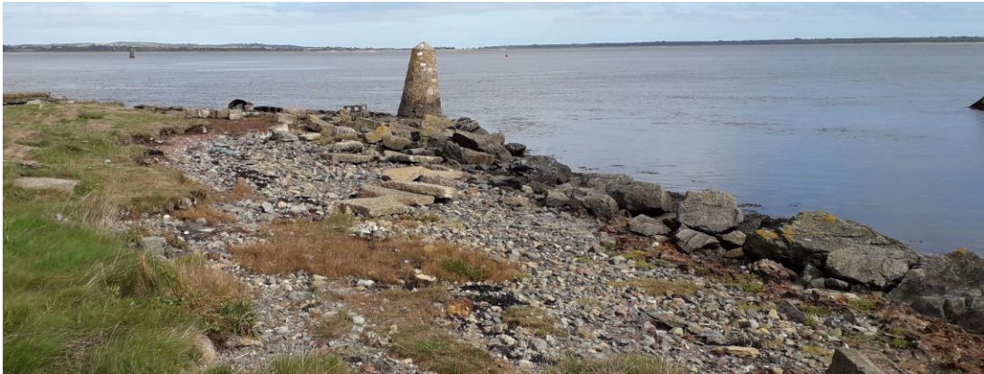
Plate 3.17 Existing sea wall facing east at the southeast corner of the site
