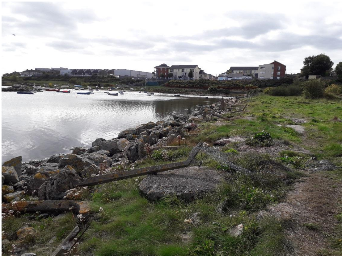
Plate 4.25 Existing Sea Wall – Southeast edge
